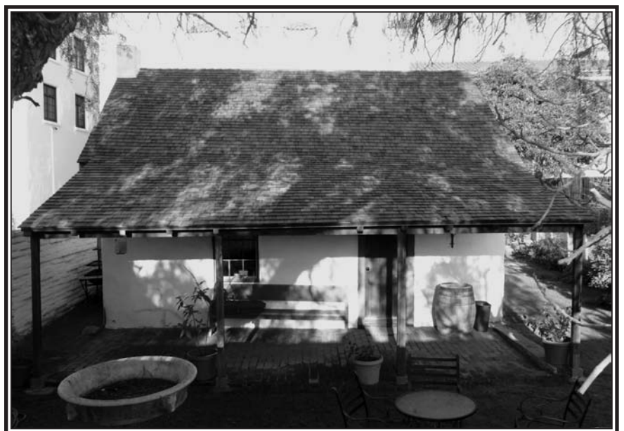
Repaired to last another 30 years.
