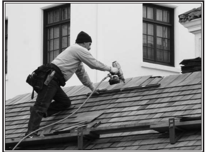
Nailing down the roof repairs.
